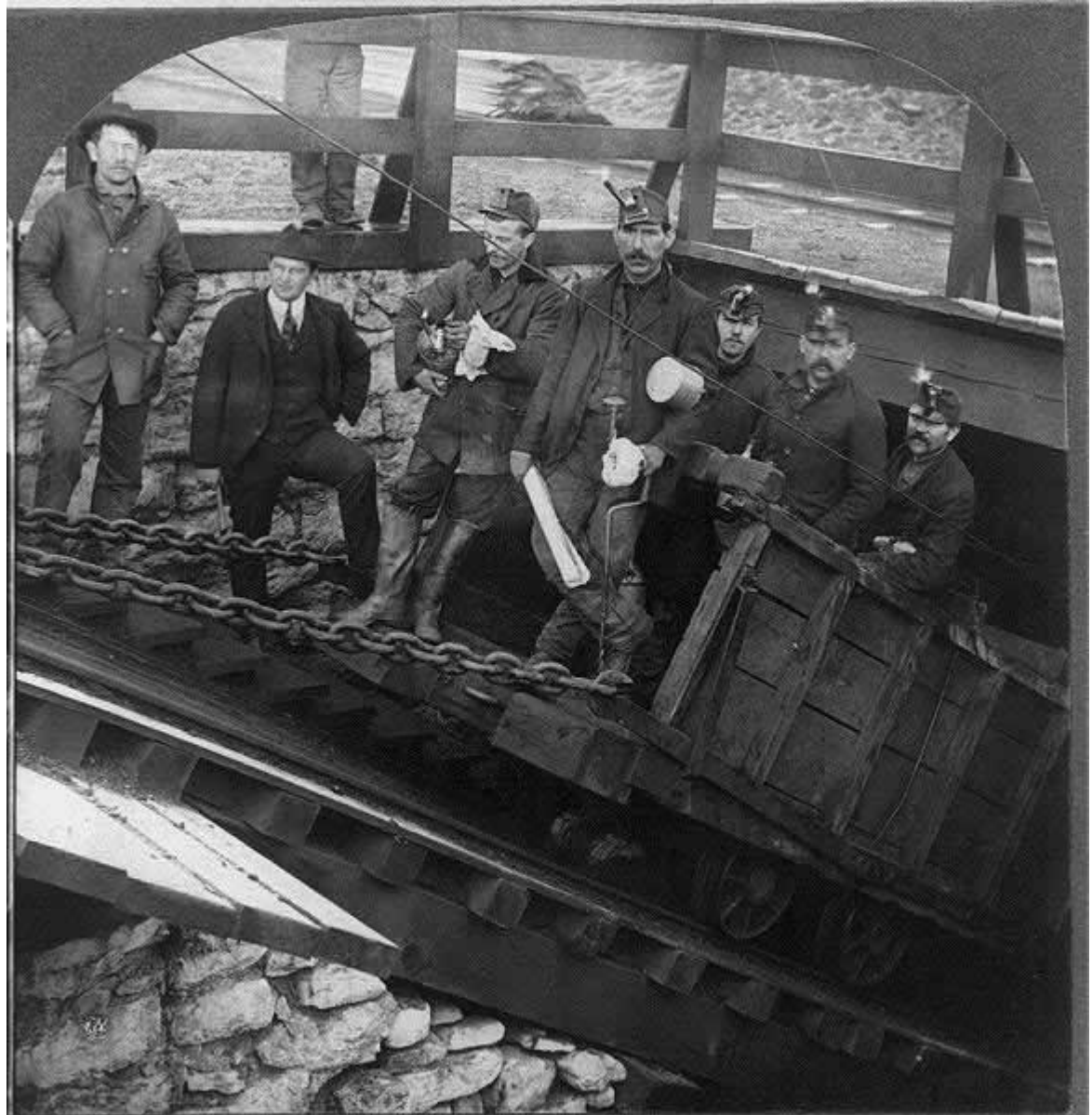
20049—Miners Going into the Slope, Hazleton, Pa., U. S. A.
